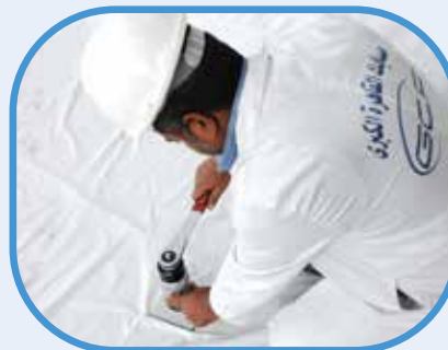
Pull Off Test
